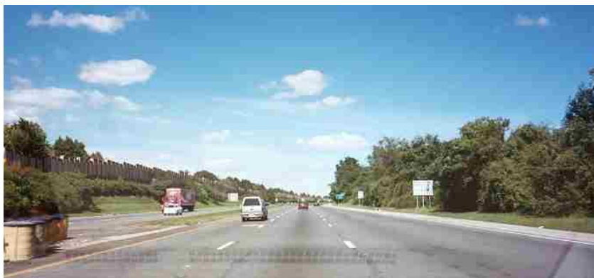
Figure IV-7 —Views of I-95 Mainline east of NJ Route 29 looking east
