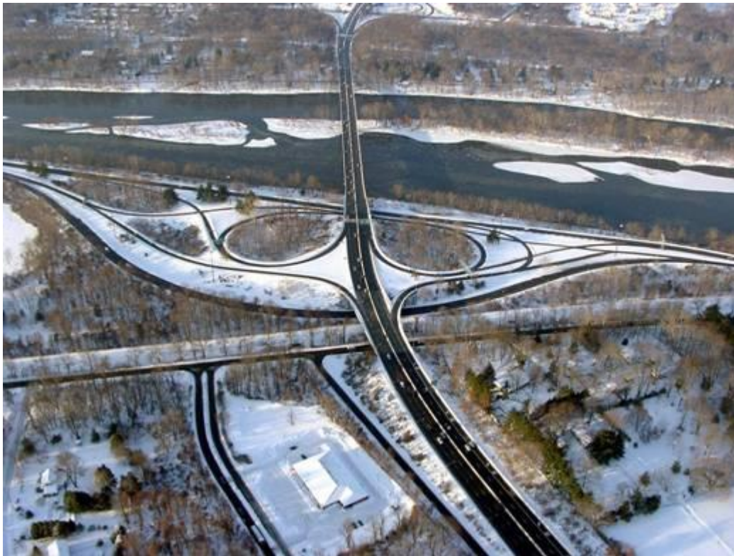
Figure I-8 —Aerial view looking west showing scissors configuration and intersecting interchange ramps at the existing NJ Route 29 Interchange
