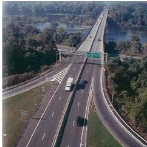
Figure I-4 —Aerial view looking south showing lack of adequate acceleration/deceleration lanes where the NJ Route 29 ramps merge/diverge at the I-95/Scudder Falls Bridge
