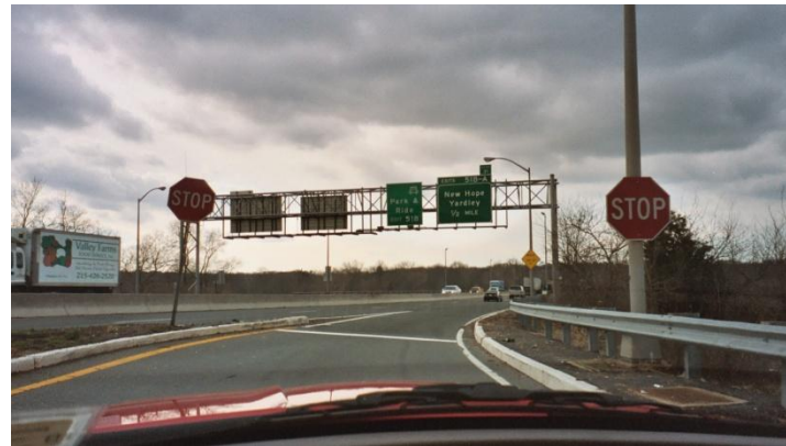
Figure I-5 —View looking south at NJ Route 29 on-ramp entry onto the I-95/Scudder Falls Bridge southbound, showing stop sign necessary due to inadequate acceleration lane
