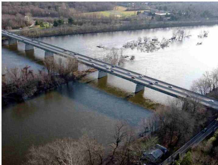
Figure IV-8 —Aerial view looking southeast at I-95/Scudder Falls Bridge
