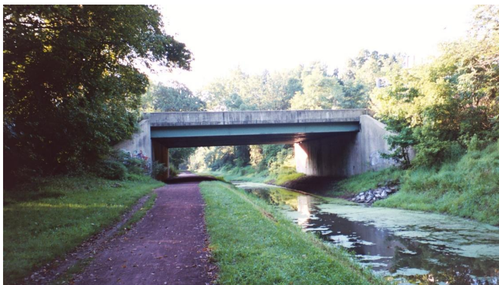
Figure IV-12—View, looking east, of I-95 Bridge over Delaware Canal
