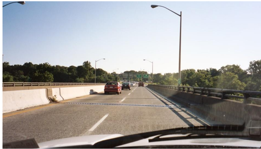
Figure I-3 —View looking northbound showing lack of shoulders on I-95/Scudder Falls Bridge
